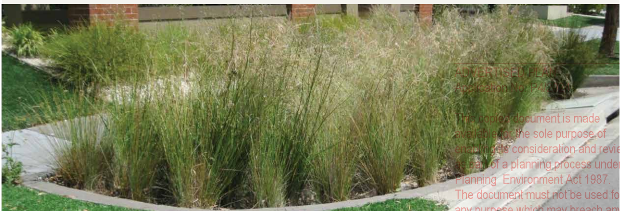
Figure 5 Healthy, densely planted vegetation is important to the long term performance of the raingarden
