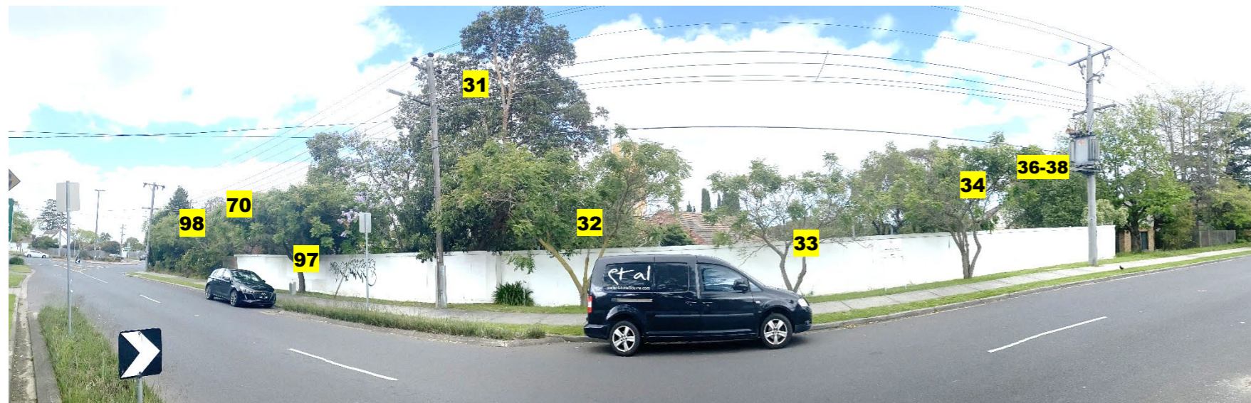
Image 2: Maltravers Rd frontage.
