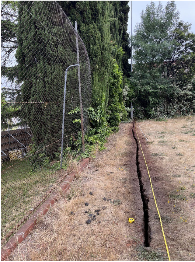
Image 12: Trench adjacent to Trees 12-16
