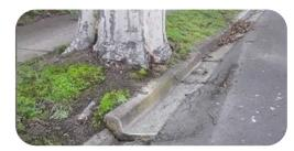
Figure 11. Poor soil depth, small planting footprint and compacted soils cause damage to footpaths. Source: Banyule City Council
