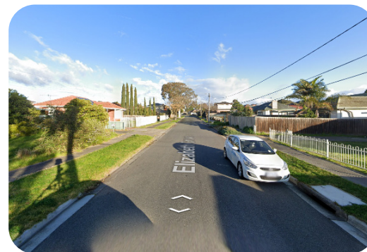
Figure 6. Streetscape view of poorly shaded footpaths in Bundoora. Source: Google Maps
