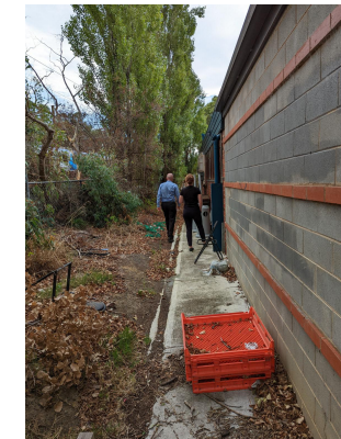
EXISTING CONDITIONS - PHOTO 12
