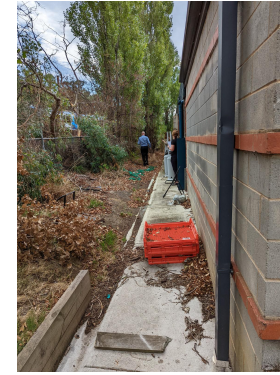
EXISTING CONDITIONS - PHOTO 4
