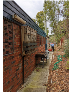
EXISTING CONDITIONS - PHOTO 3
