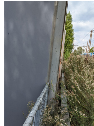
EXISTING CONDITIONS - PHOTO 11
