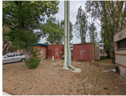
EXISTING CONDITIONS - PHOTO 2
