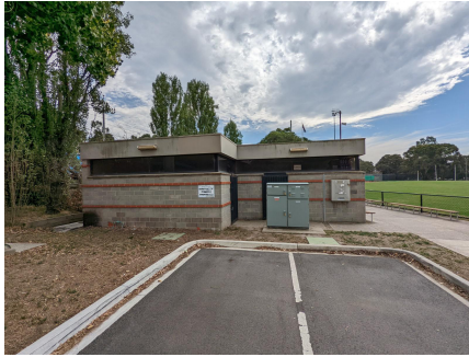
EXISTING CONDITIONS - PHOTO 1
