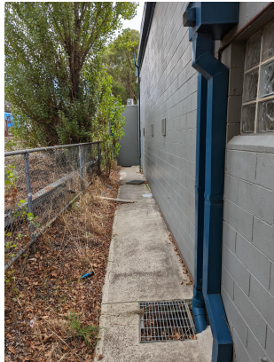
EXISTING CONDITIONS - PHOTO 5
