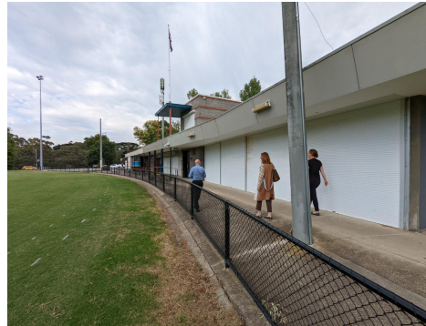
EXISTING CONDITIONS - PHOTO 7
