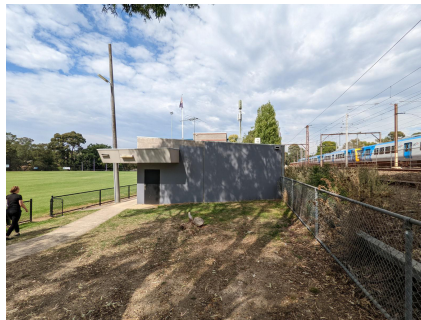
EXISTING CONDITIONS - PHOTO 9
