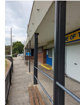
EXISTING CONDITIONS - PHOTO 8
