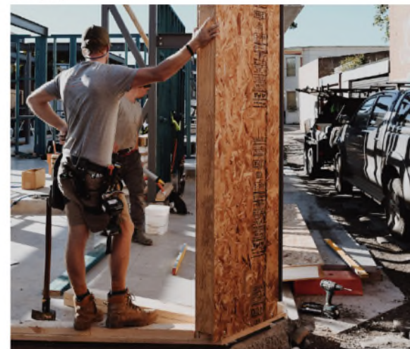
Construction site of townhouse development. Photography by Sunlyt Studios
