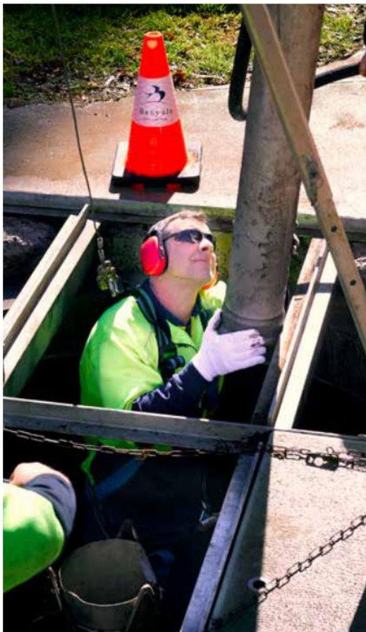
Removing waste from the gross pollutants trap at Chelsworth Park
