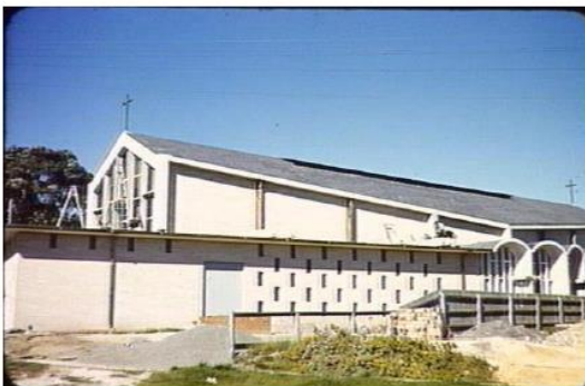
View to west elevation, during construction – note barrel vaulting (Source: Peter Wille, undated, SLV, no a22359)
