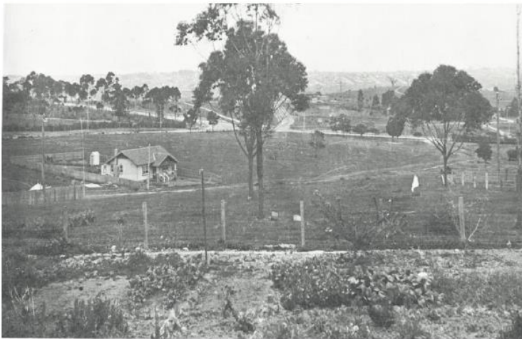
Late 1920s photograph across Ivanhoe East from Maltravers Road with the junction of Lower Heidelberg and McArthur roads (East Ivanhoe Village) visible in the centre – Mother of God Church would be constructed out of frame left. (Source: Cyril Cummins, A pictorial history of Heidelberg Since 1836 , Heidelberg Historical Society, 1982, p71)
