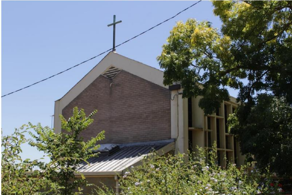
South (rear) elevation with later addition skillion volume in the foreground and section of window wall with 'random' mutin bars on right of frame
