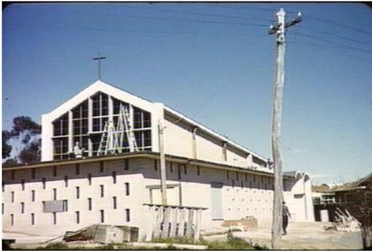
View to frontage and along west elevation, during construction (Source: Peter Wille, undated, SLV, no a22359)
