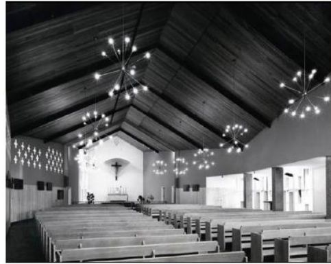
Original nave showing 'starburst' light fittings (replaced) and steel beams (Source: www.ivanhoecatholics.com/parishhistory.htm )
