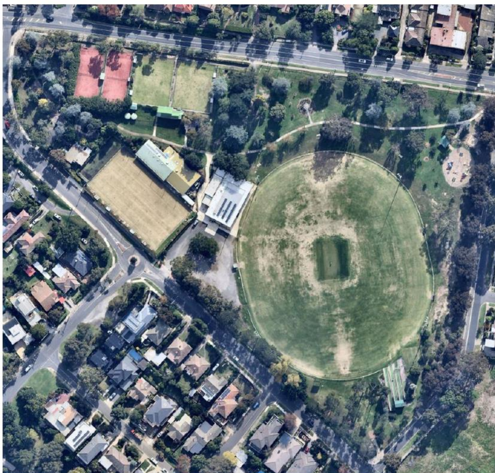
Figure 5: Aerial View of Ivanhoe Park
