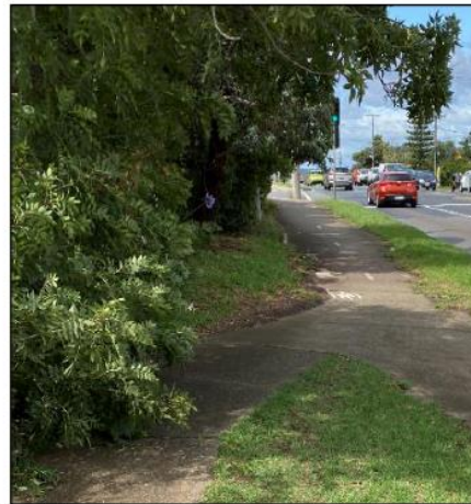
Off-road shared path (Greensborough Road) – Northbound route ends abruptly
