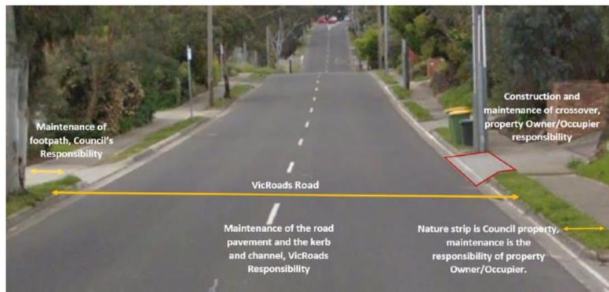
Figure 2. Operational Responsibility on Arterial Roads
