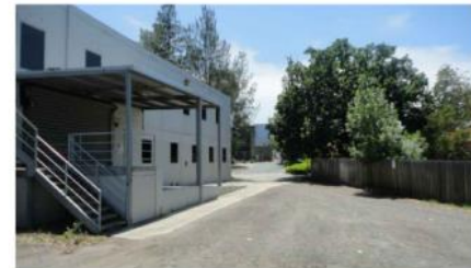
7. View from within site looking West.
