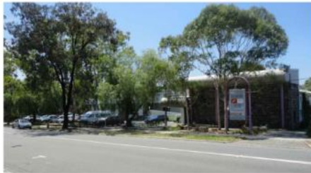
2. Adjoining property to South of subject site on Turnham Ave, looking North East.
