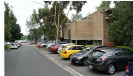
4. Douglas Street looking South through rear of site.
