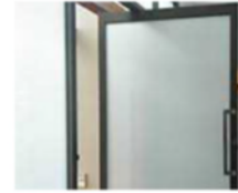
015 - aluminium framed windows with frosted glass Powder coat finish (black) - colour to be confirmed
