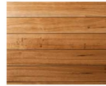
018 - Existing - weathered pine or treated pine cladding
