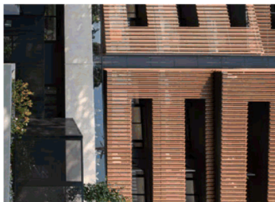
TIMBER LOOK ALUMINIUM FINNS TO EXTERNAL FACADE SKIN ACTS AS AN OUTER LAYER OF PRIVACY FOR THE APARTMENTS
