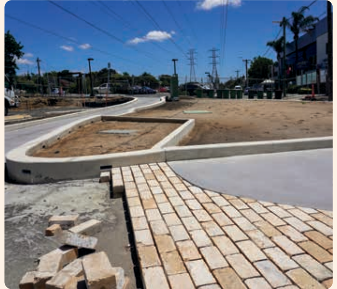
Landscaping work underway near Morwell Avenue
