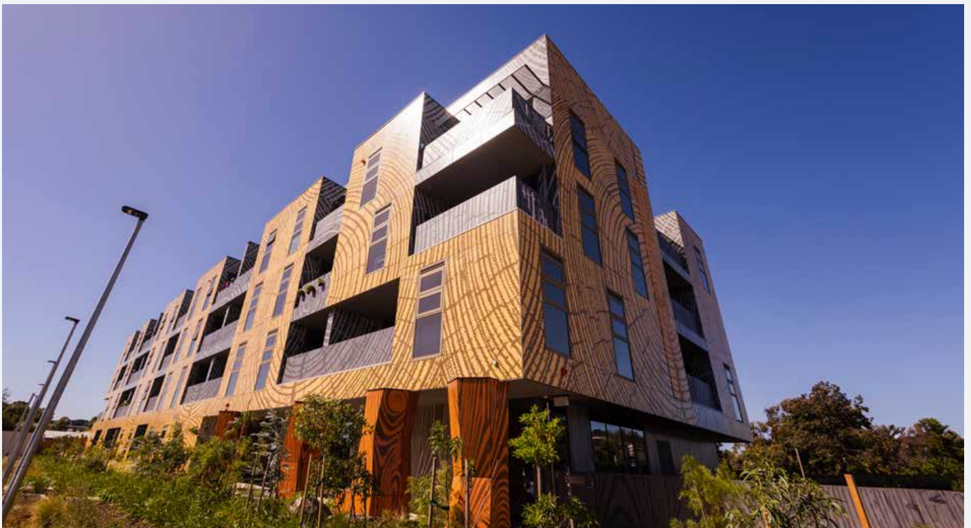
Bellfield Social Housing Development
