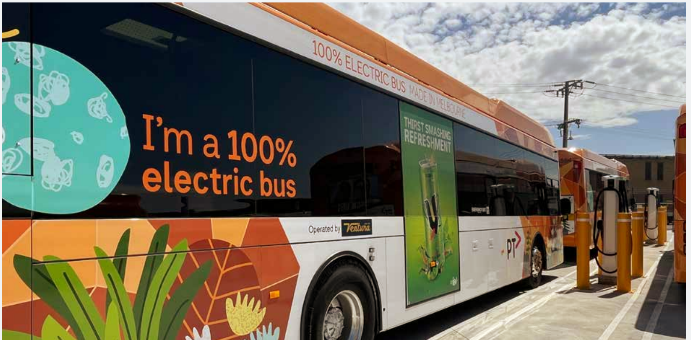
Ventura Electric Bus Depot, HWBP
