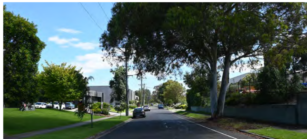
Sheehan Road streetscape
