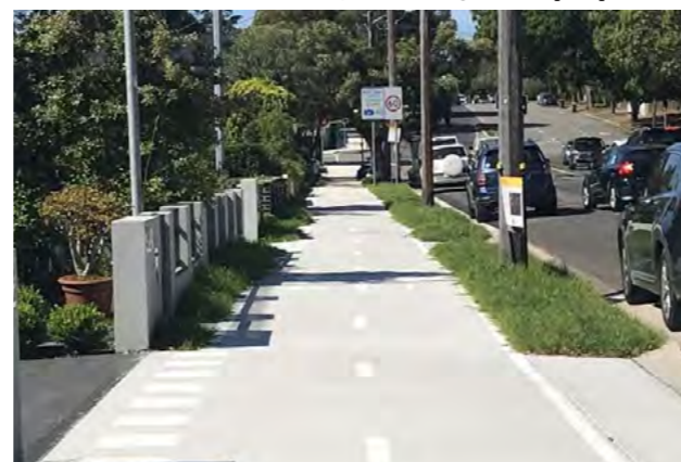
Interface safely with adjacent properties
