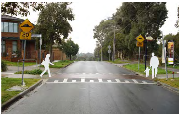
Raised pavement pedestrian crossing in Heidelberg.
