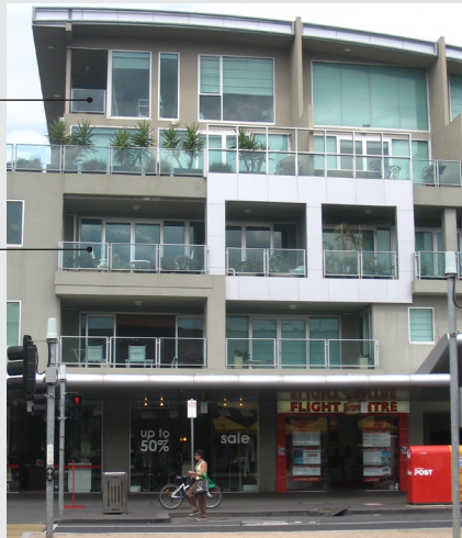
Buildings with a 3 storey façade showing upper levels set back and balconies recessed into the third storey.
