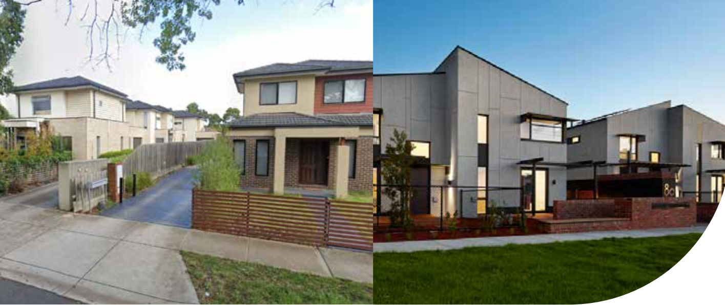
Figure 11: Left: Infill development on individual suburban lots: note the duplication of driveways resulting in reduced open space, increased impervious surfaces and limited flexibility in dwelling siting. Right: Infill development on two-lot consolidation: Greater flexibility is provided to explore more innovative landscape planning and access arrangements, improved landscape outcomes with no loss in dwelling yield.
