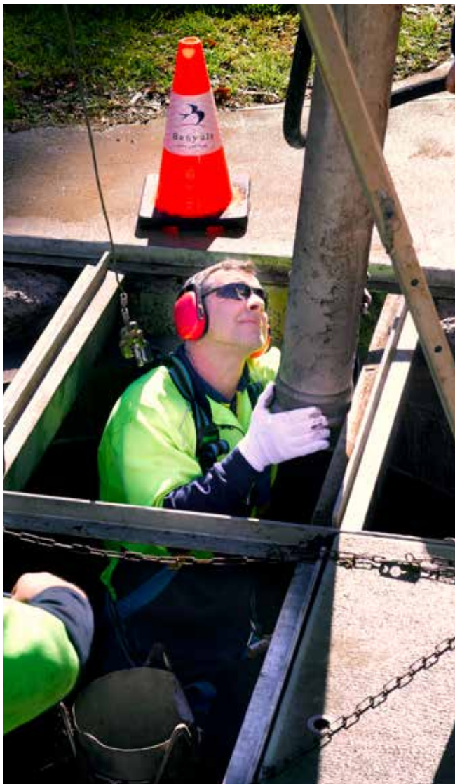
Removing waste from the gross pollutant trap at Chelsworth Park
