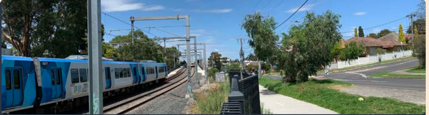
Alongside the Hurstbridge rail corridor near Rosanna station.
