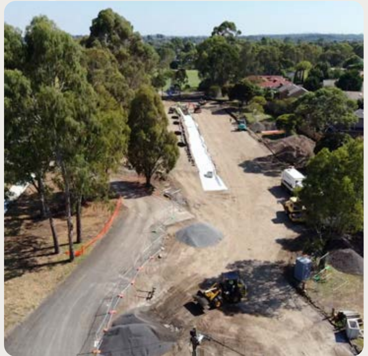
A new car park under construction (Stage 3).
