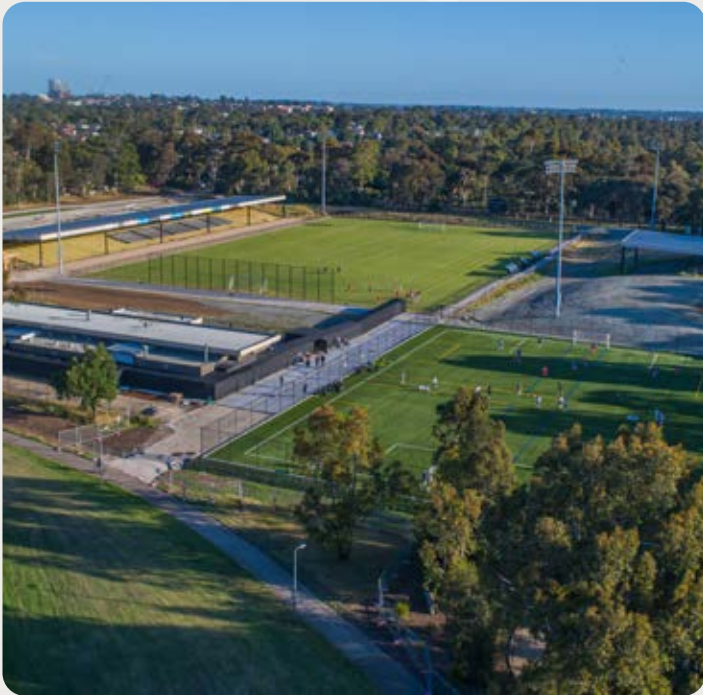
The new main pitch (top left) and synthetic mini-roos soccer pitch (right).
