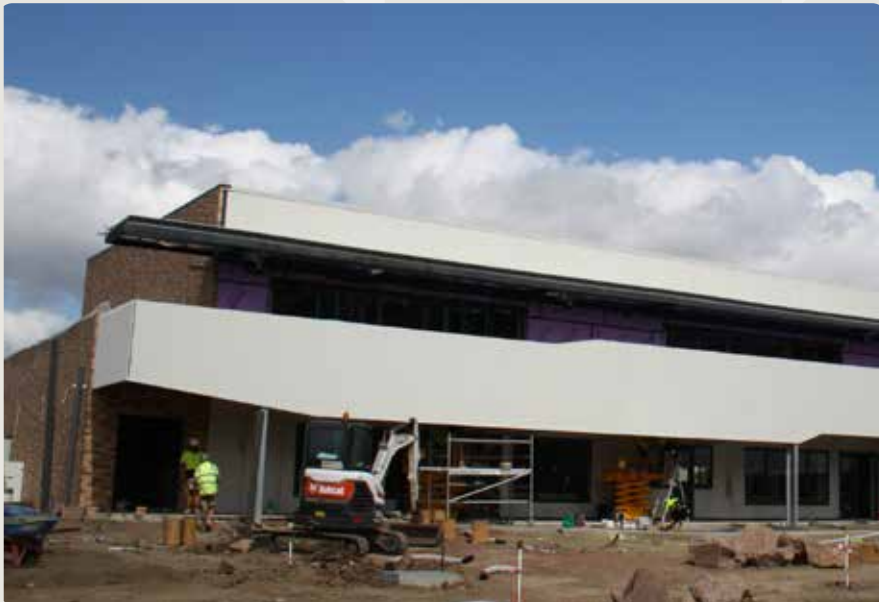
Bellfield Community Hub under construction 1 April 2022.
