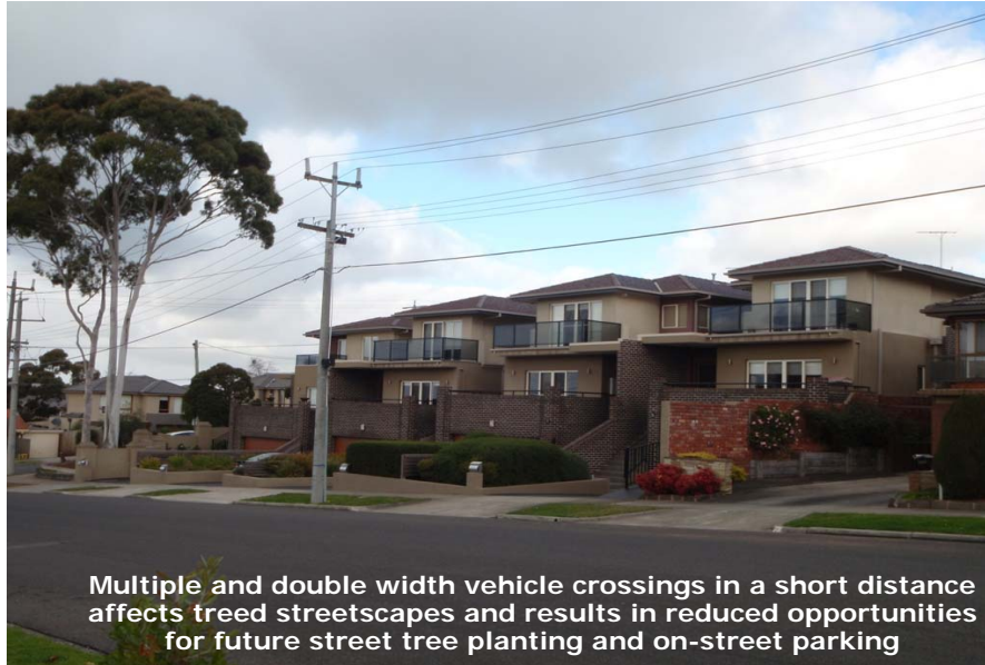
Figure 3: Multiple and double width vehicle crossings in a short distance
