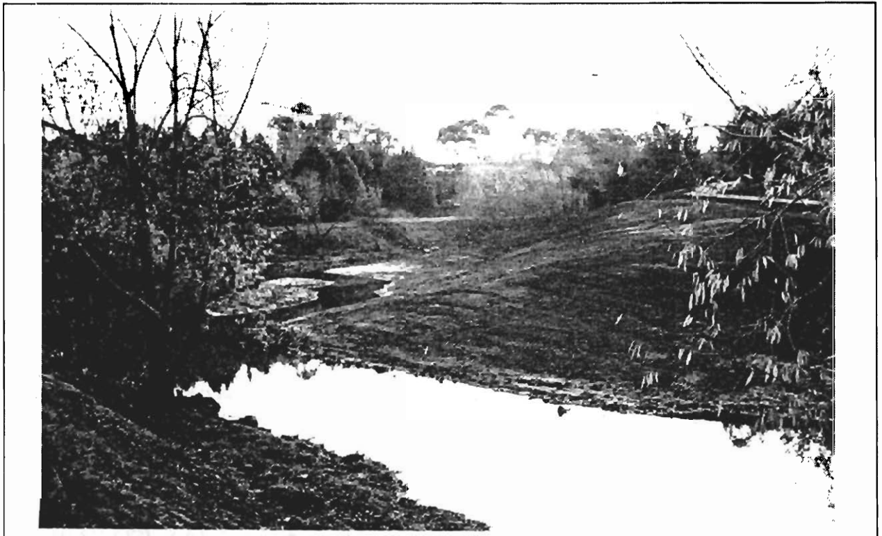
Photo 8: Recently completed wetlands project north of Banksia Street
