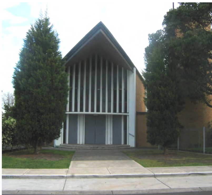
St Bernadette's Catholic Church, Bond Street, Ivanhoe.
