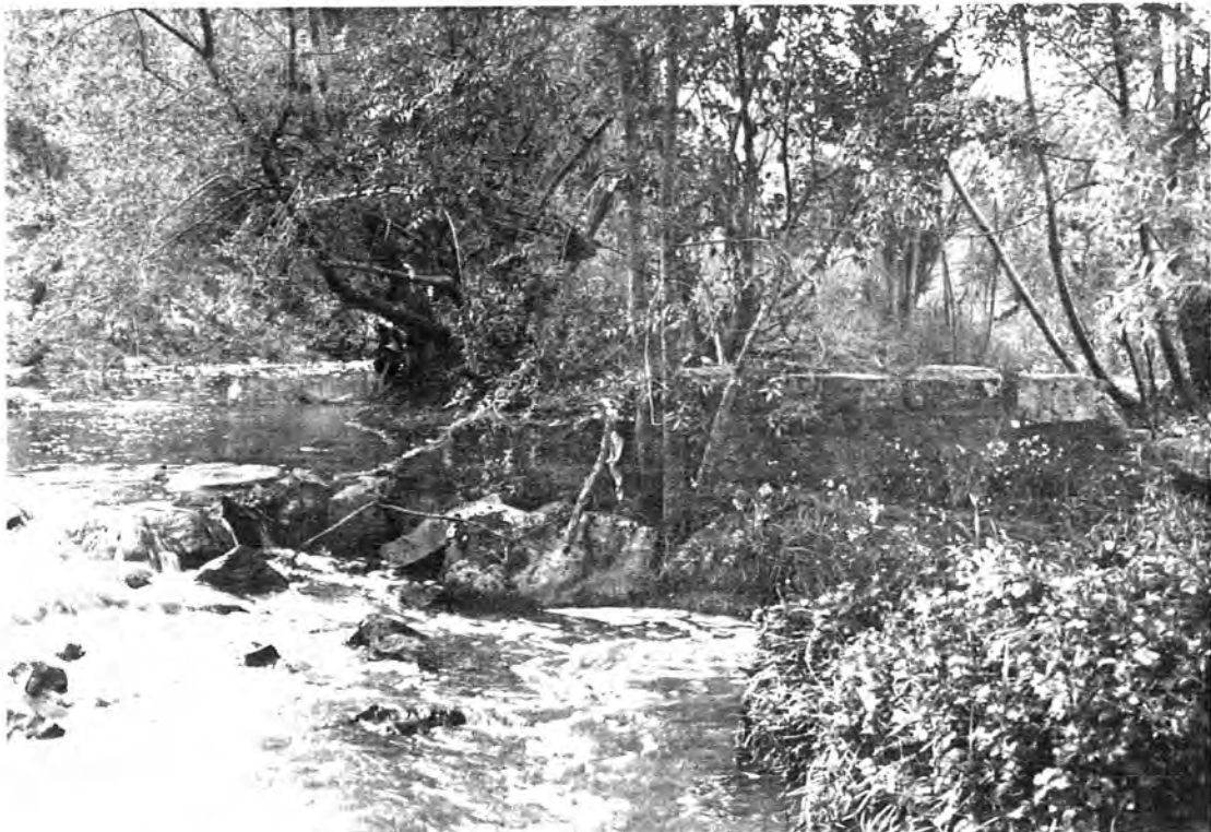
WEIR WALL — DAREBIN PARK
