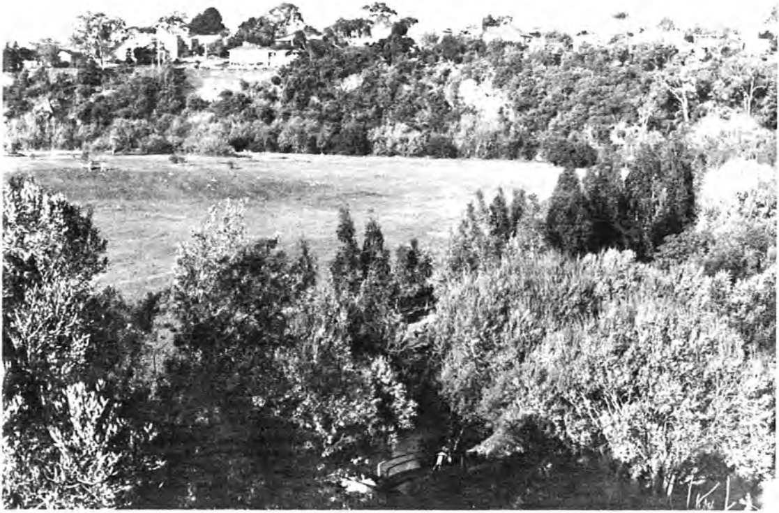
DAREBIN PARKLAND VIEW TO THE NORTH
